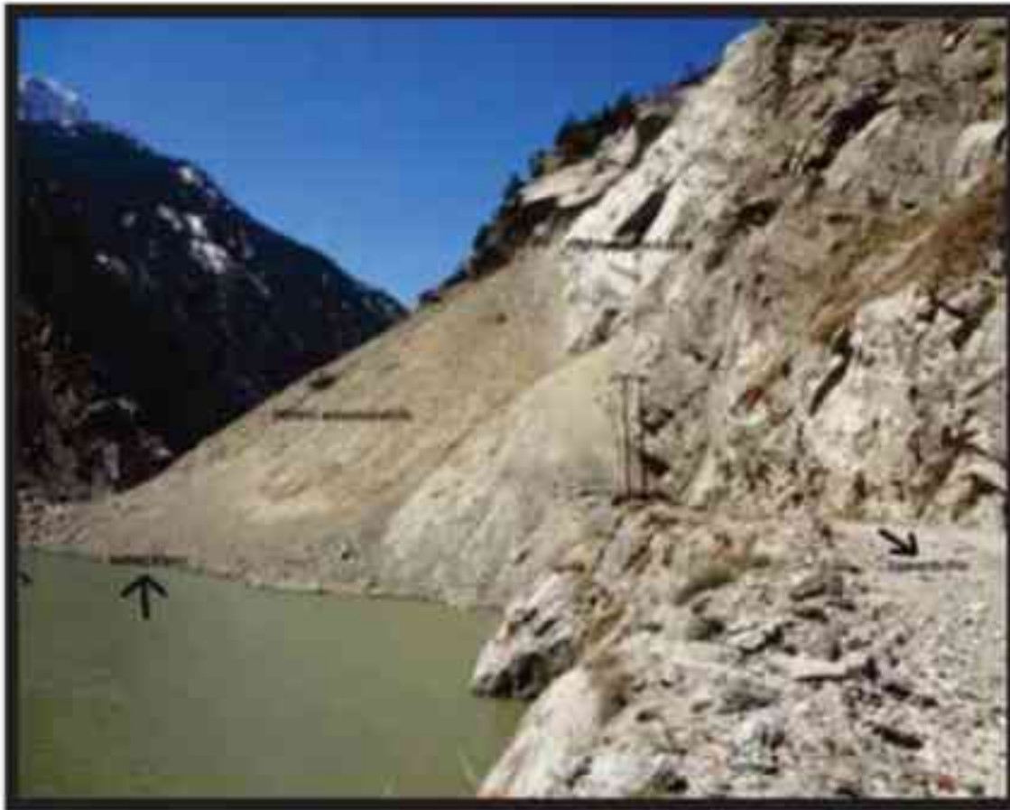
Debris cone over road and river
