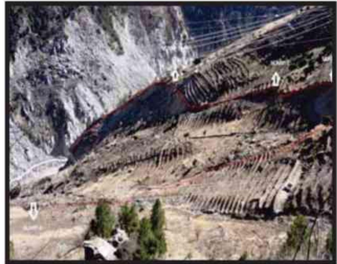
View of Urni landslide
