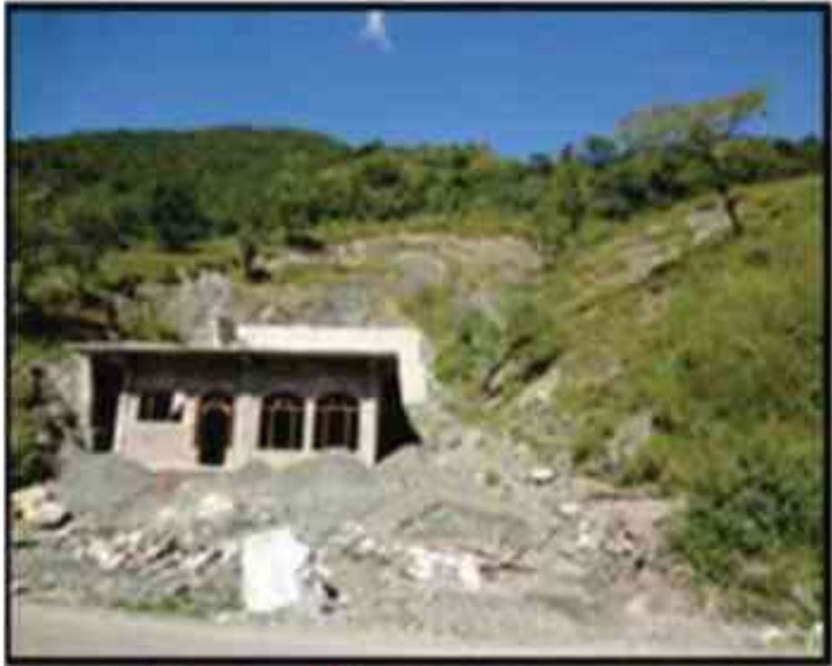
Debris slide near Chirang, NH-20, Mandi
