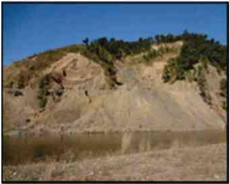
Debris slide near Dadahu, Sirmur
