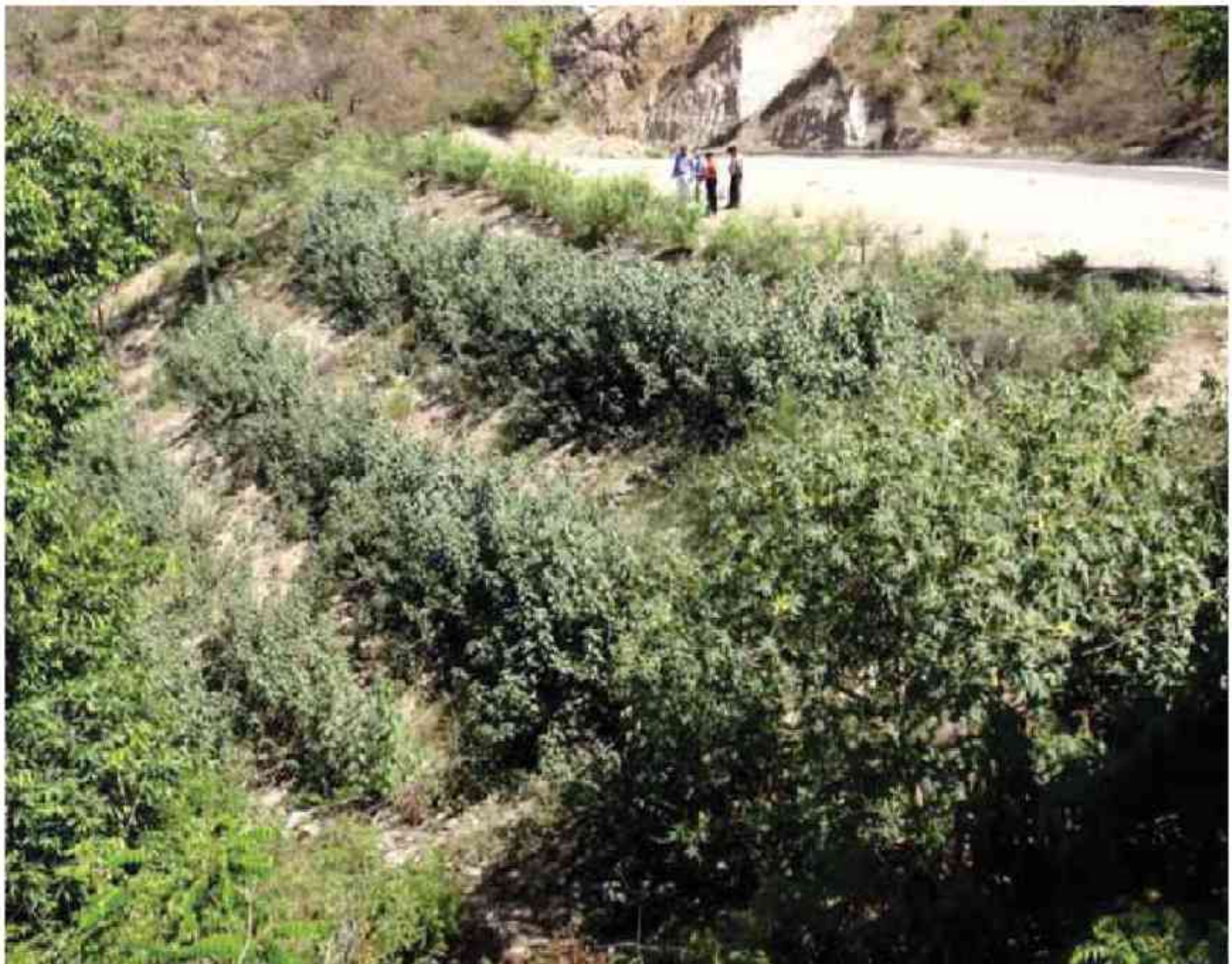
Slope Stabilization through Bio-engineering
