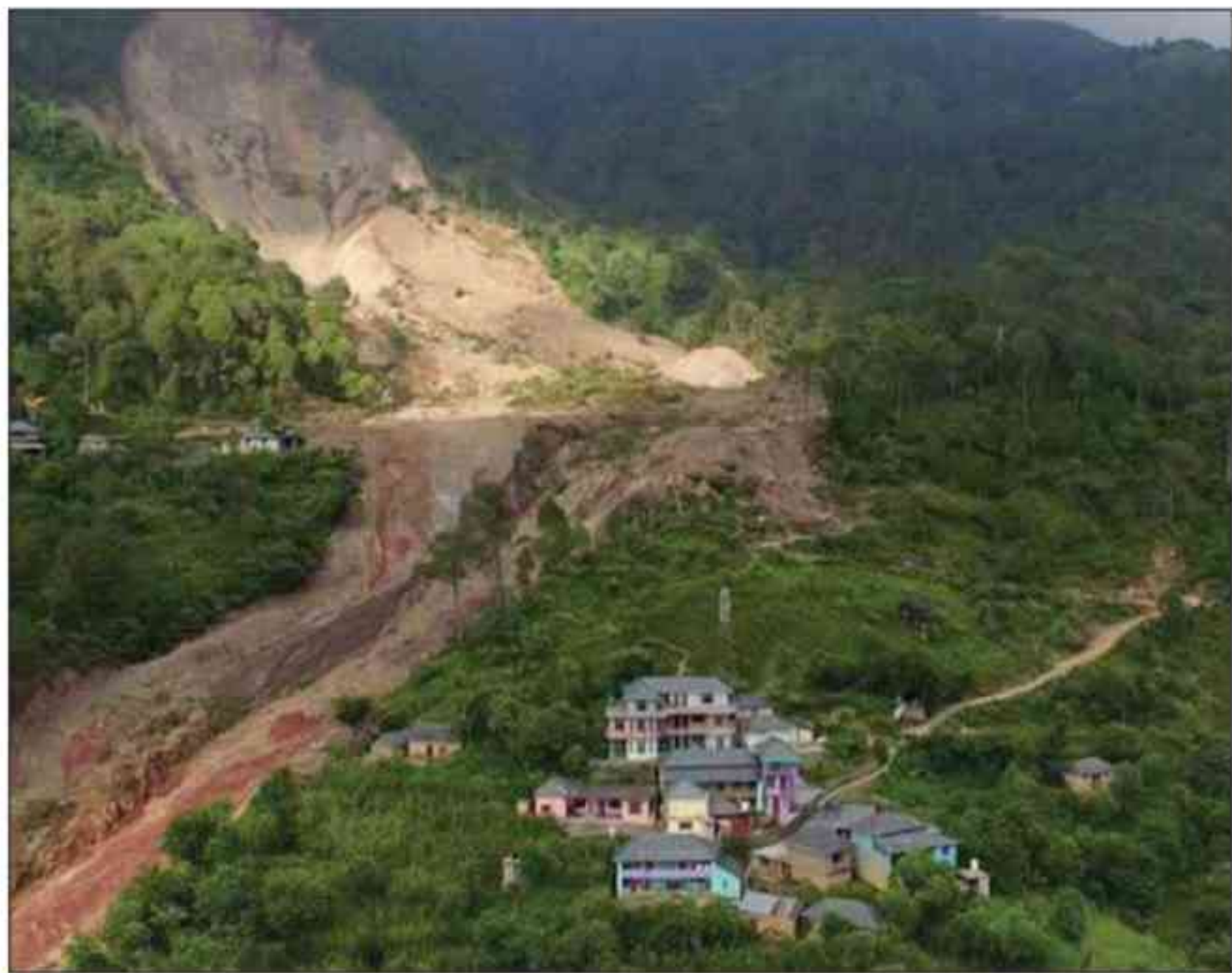
Field Photograph of Kotrupi Landslide
